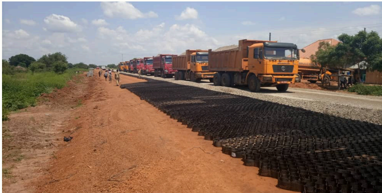
7. Finished & Compacted Base Layer
