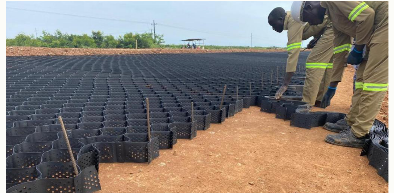
4. Installation of PRS Neoloy Tough Cells Sub Base Layer
