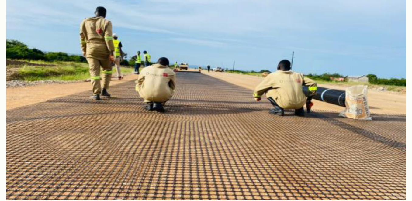
2. Pioneer layer Preparation+Installation of Geogrid Upper Subgrade Layer
