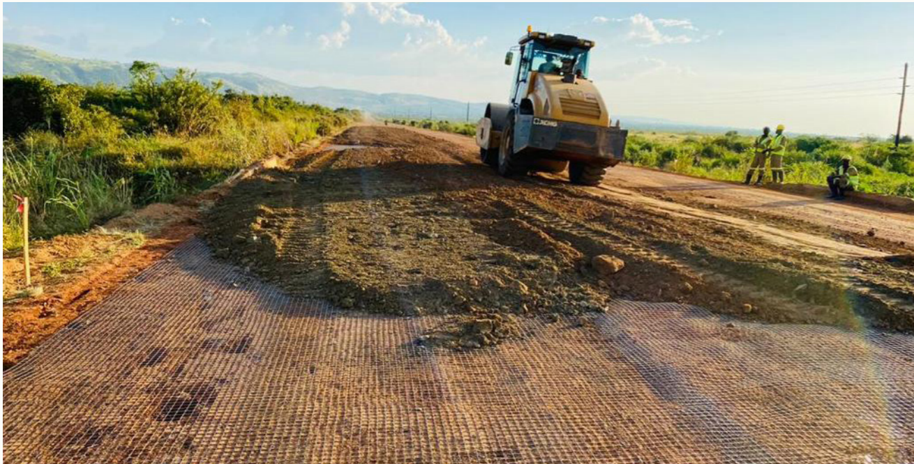
3. Fill Material and compaction on top of geogrid
