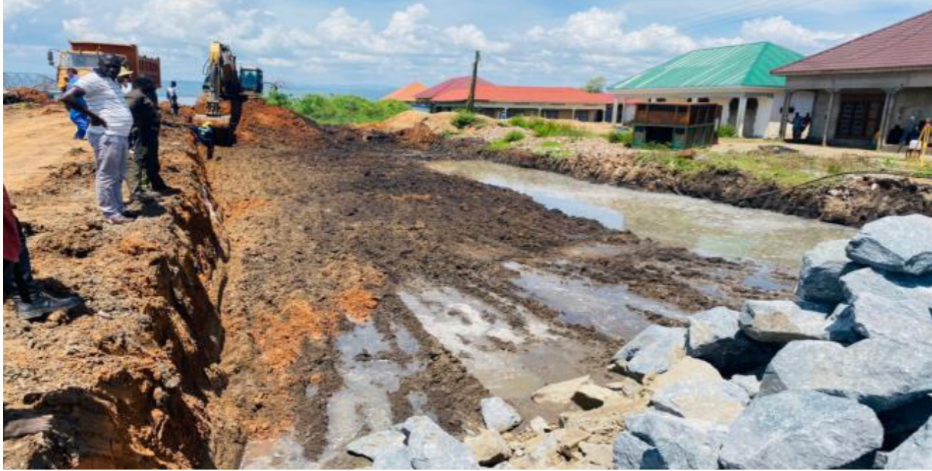
1. Existing Subgrade Condition
