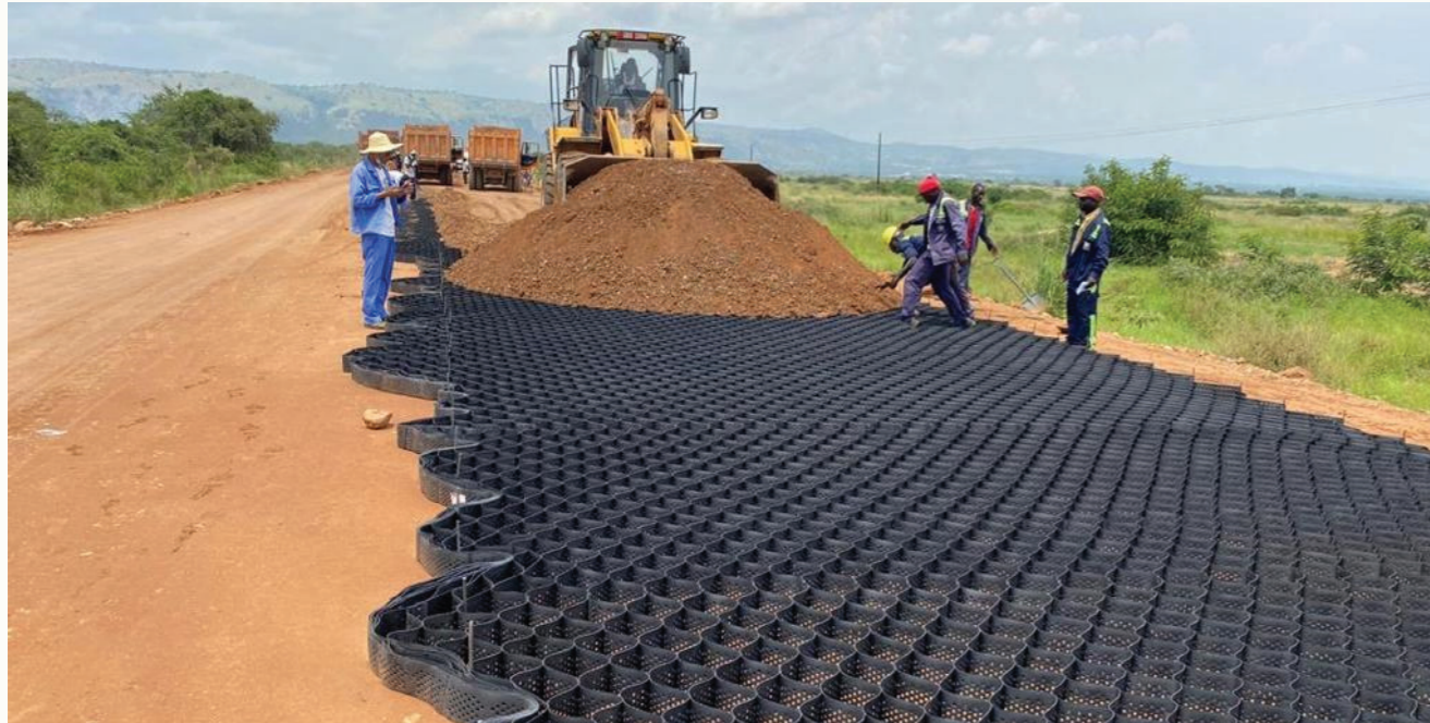
5. Fill Material Over Neoloy Tough Cells
