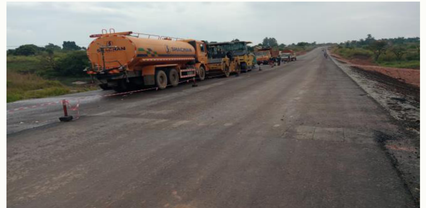
8. Installation of Final Asphalt Layer
