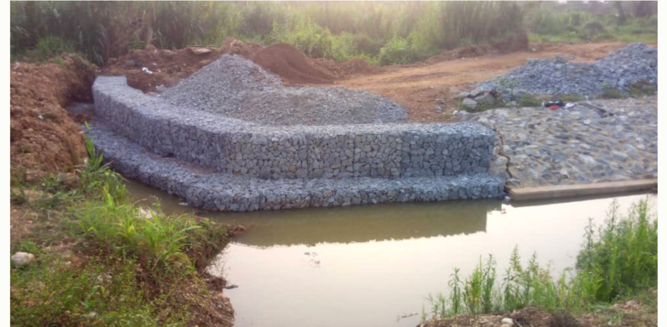
3. Completed gabion wall
