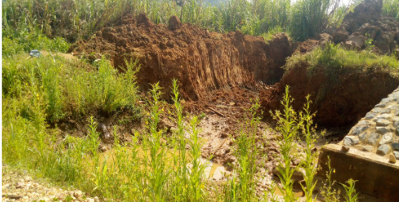
1. Excavation and ground preparation
