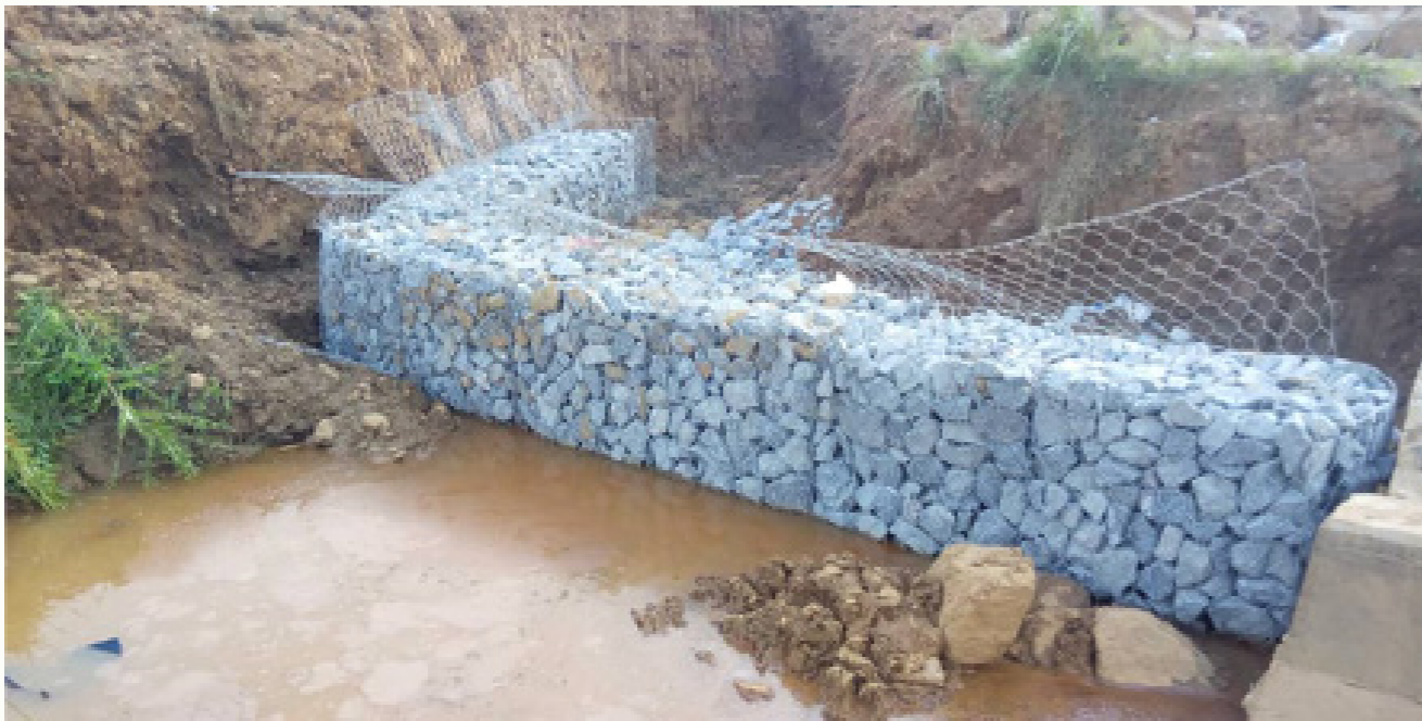
2. Placement of boulders in gabion basket
