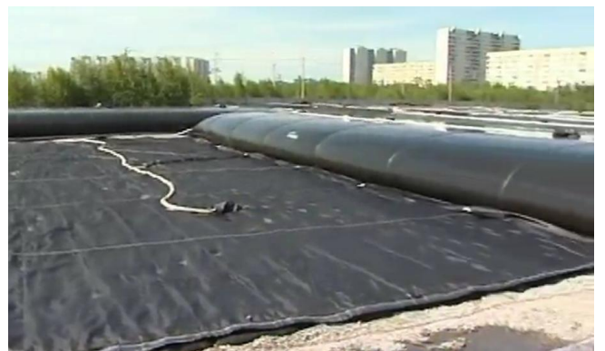
The Geotubes remained in place for continued dewatering during the winter
