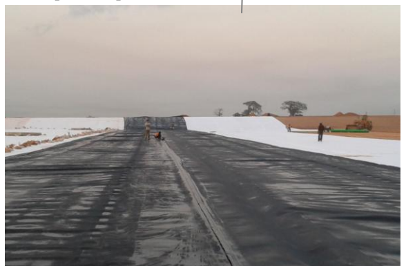
Welding of the geomembranes
