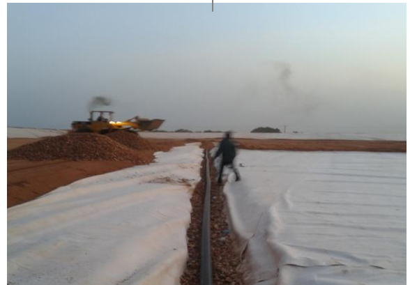
Lining of drainage channel
