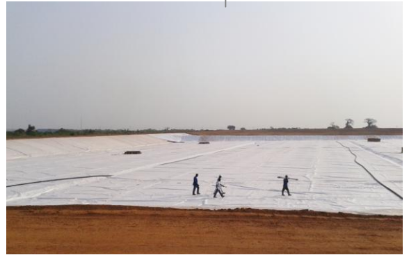
Lining of drainage channel
